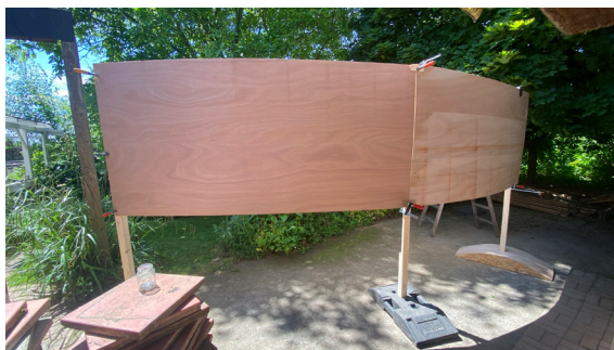
building-process of the spatial installation
